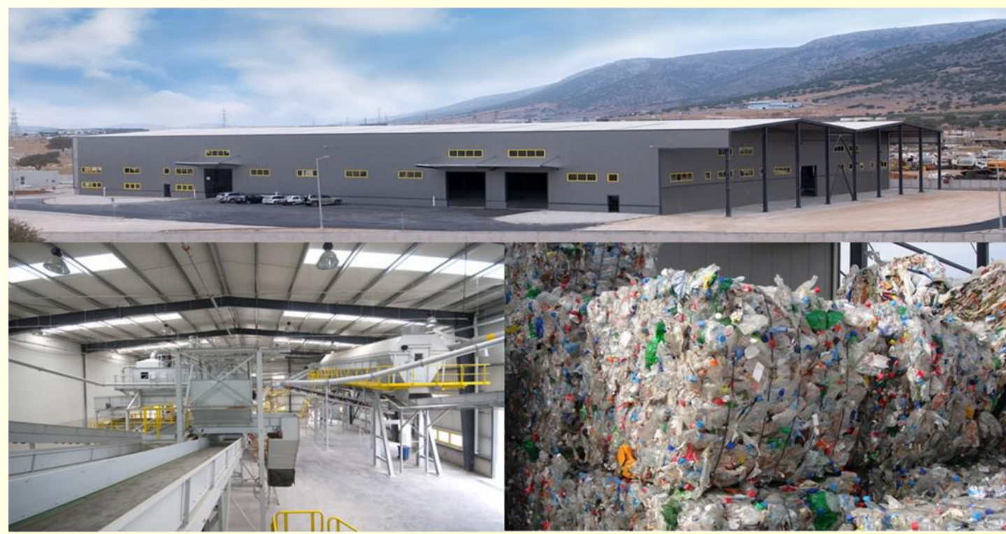
EPANA SA, Ano Liosia - MRF facility, external and internal view
